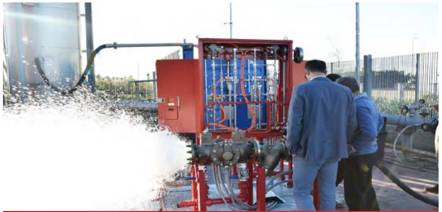
The VDD has been designed to comply with the requirement of S001 granting continuous operability even during maintenance
